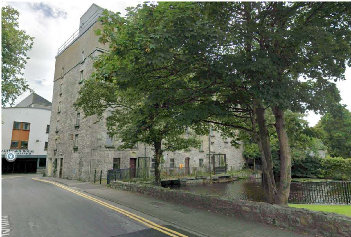
Photo 1.2 Site Access from external walkway on the North of the existing building
