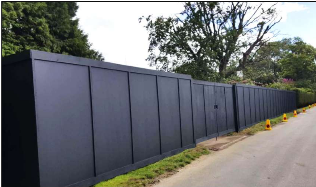
Photo 7.1: Typical Site Hoarding Arrangement
