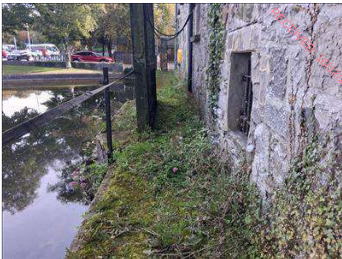
Plate 3-2 Walkway at the northern façade of the McLaughlin Building (ED3)
