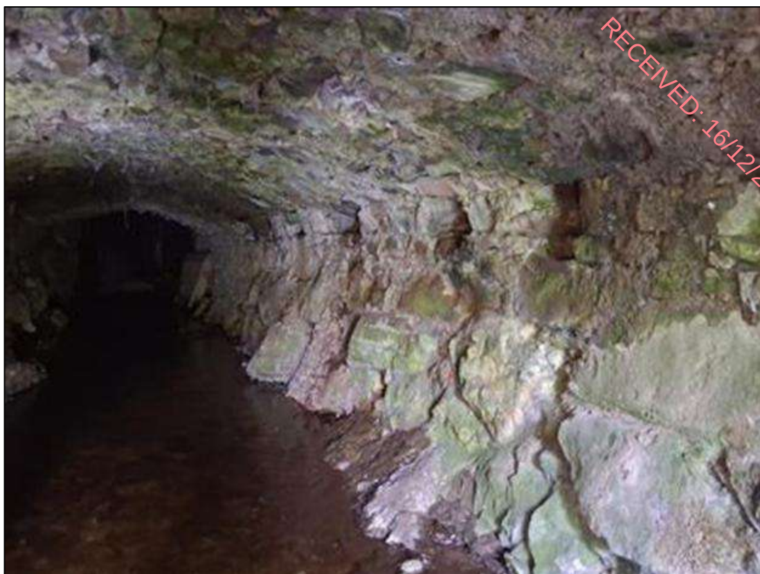
Plate 3-4 Culvert (BL1) under the McLaughlin Building
